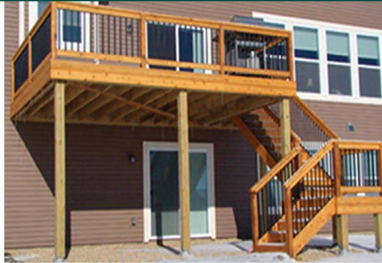
were conducted on isolated posts without railing,” Truckner explained. “Often, a continuous rail is used, which can help to distribute the load to other posts, decreasing the load effects on the bolts at a single post attachment. However, the test was designed for worst case scenarios, which were correctly reflected in the above testing.”
